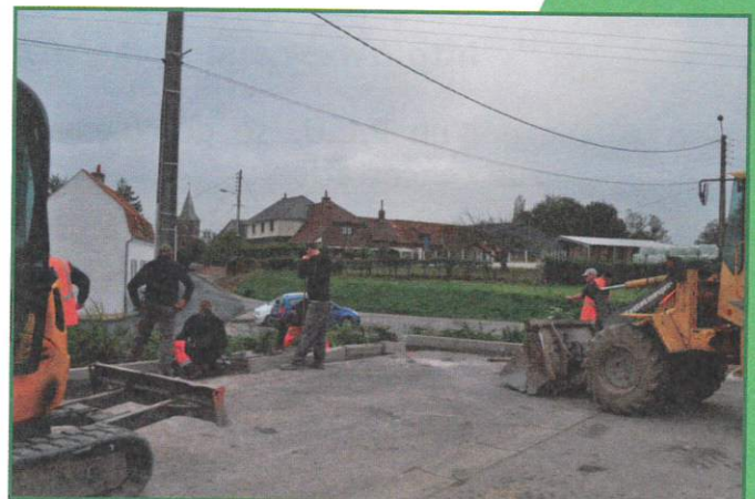
REFECTION DU PARKING A MARTHES
