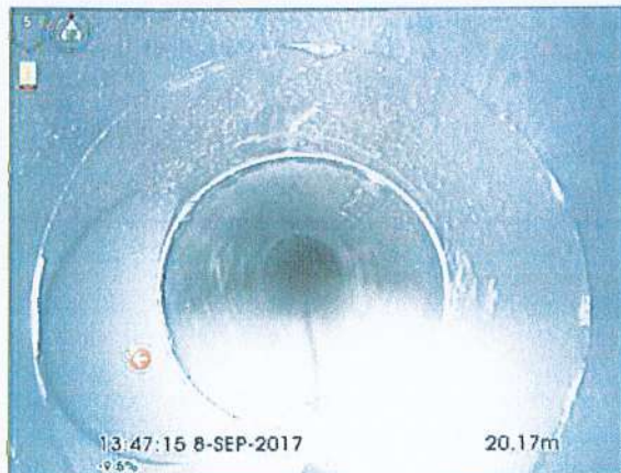
Photo: 3_3_7_A.BMP 21m, Raccordement direct à 09 h.
