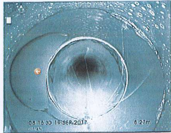
Photo: 5_5_32_A.BMP 8,5m, Raccordement direct à 10 h.
