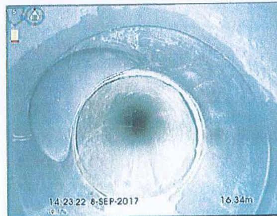
Photo: 8_8_18_A.BMP 16,6m, Raccordement direct à 10 h.
