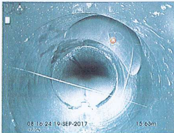
Photo: 5_5_33_A.BMP 16m, Raccordement direct à 01 h.
