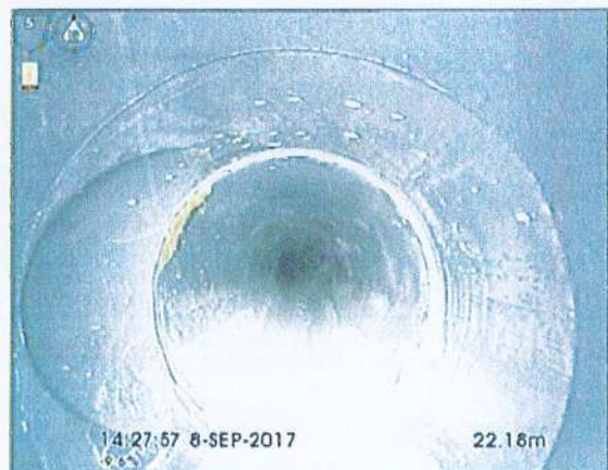
Photo: 9_9_23_A.BMP 22,6m, Raccordement direct à 09 h.
