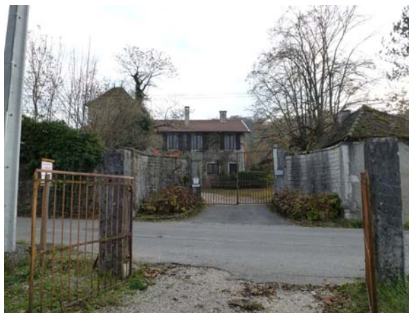
Construction au Village
