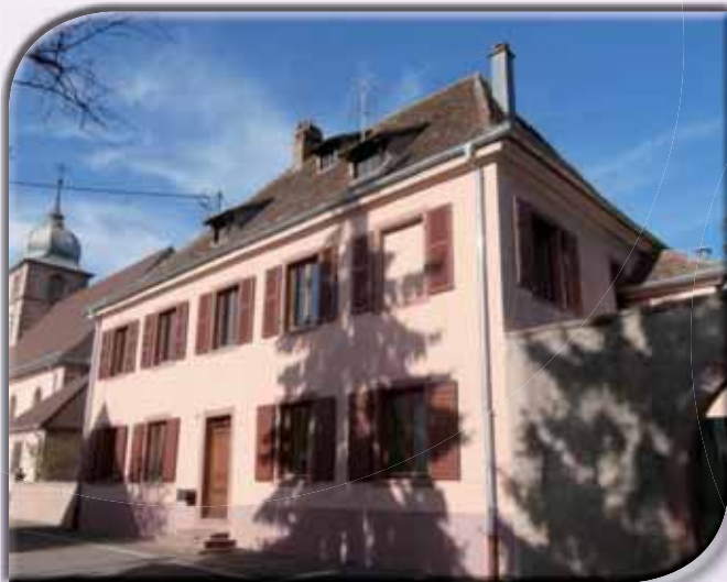
RENOVATION DU PRESBYTERE
