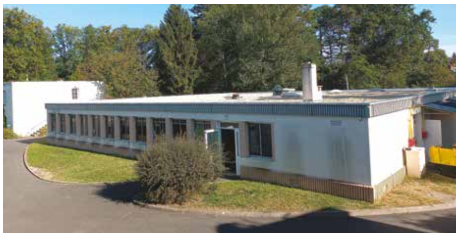
Restaurant scolaire Beaumer
