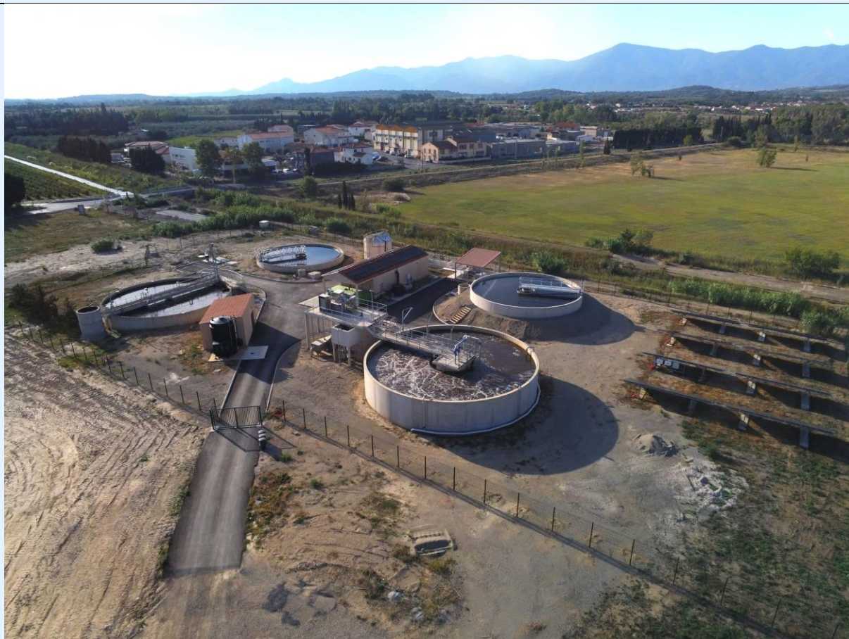
Extension station d'épuration - Bages
