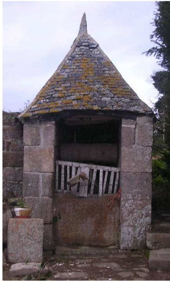
1- Puits Village de Pors Royal
