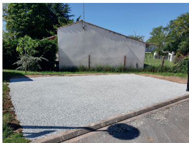
Parking Hauts de Lormont
