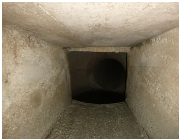
Exutoire pluvial (750x720mm)
