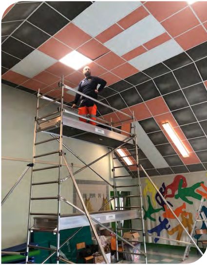
Installation d'éclairage LED.
