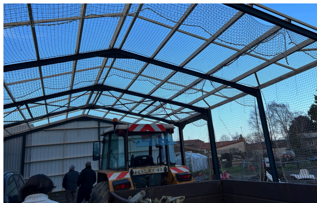
Extension atelier technique - rue Gustave Eiffel
