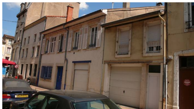
Percements de garages
