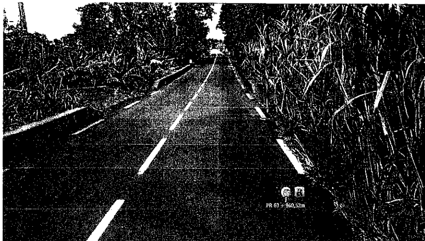
Identification: Images Avant Date: 13/04/2015 Localisation : 974 N0002(+) PR 63 + 959,52m; PR 64 - 58,18m
