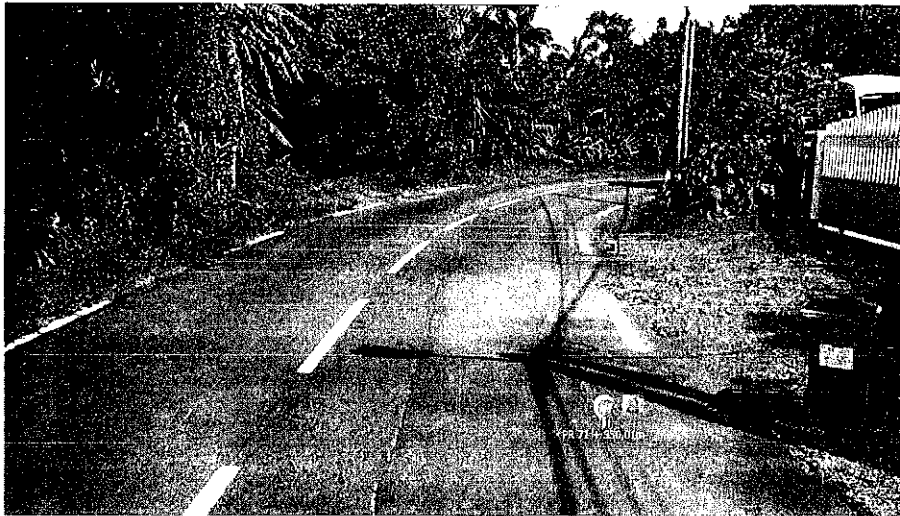
Identification: Images Avant Date: 13/04/2015 Localisation : 974 N0002(+) PR 71 + 949,01m; PR 72 - 41,59m
