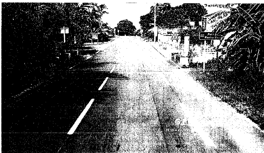
Identification: Images Avant Date: 13/04/2015 Localisation : 974 N0002(+) PR 58 + 433,50m; PR 59 - 577,61m
