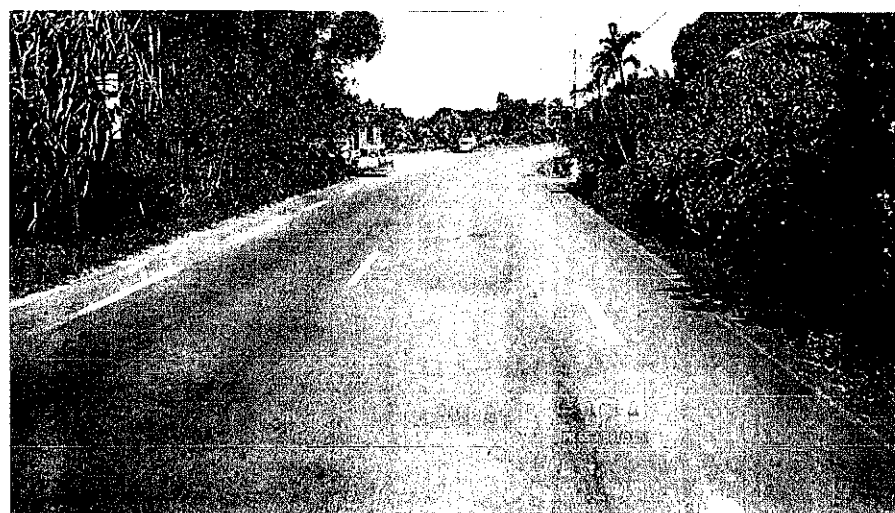
Identification: Images Avant Date: 13/04/2015 Localisation : 974 N0002(+) PR 65 + 380,33m; PR 66 - 626,22m
