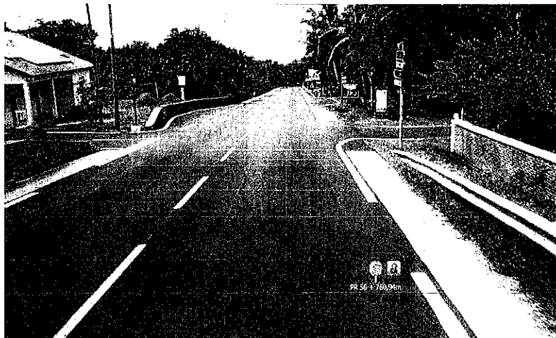
Identification: Images Avant Date: 13/04/2015 Localisation : 974 N0002(+)-PR 56 + 759,94m; PR 57 - 314,22m
