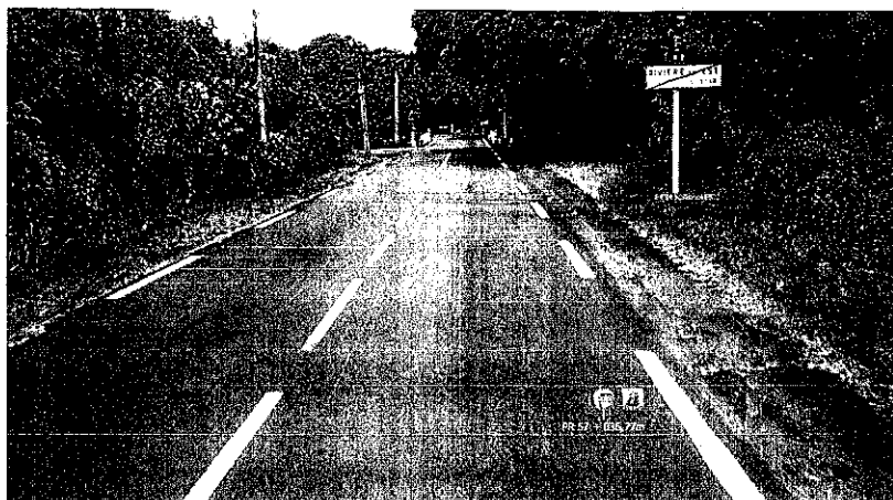
Identification: Images Avant Date: 13/04/2015 Localisation : 974 N0002(+) PR 57 + 835,77m; PR 58 - 161,53m
